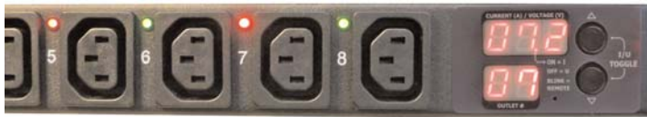
Rear of 1U PDU showing current draw for outlet #7. Red LEDs show outlets that are switched on. Green LEDs show outlets that are switched off.
